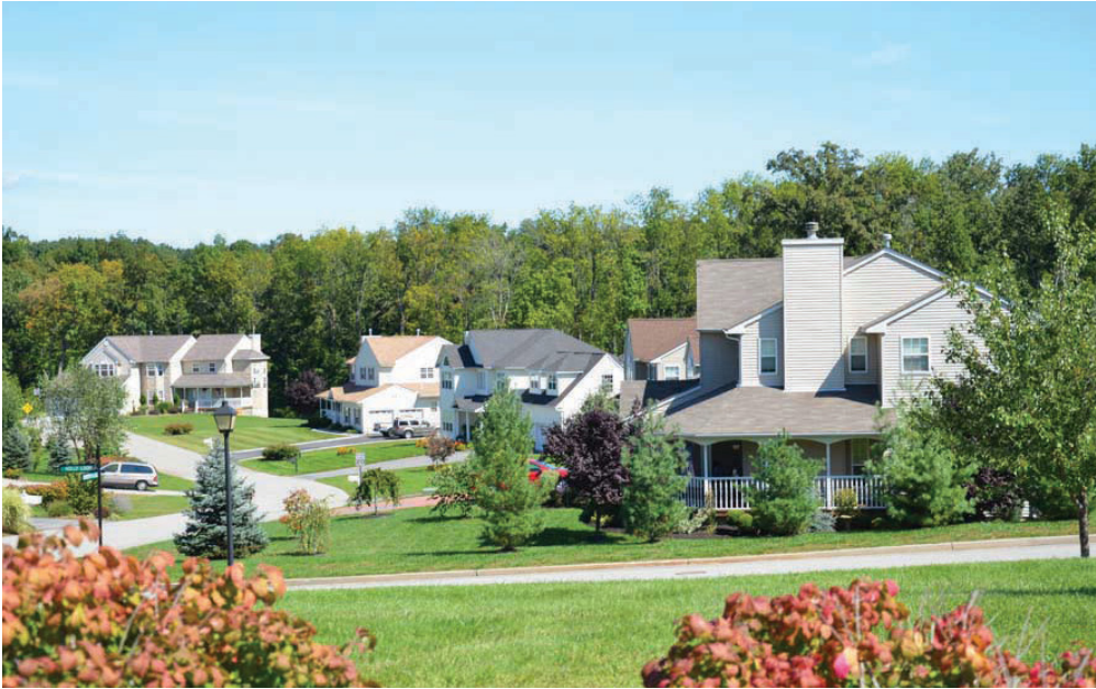
Credit: AVR Homebuilders
