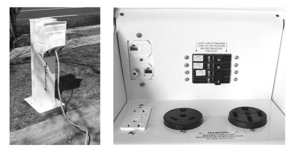
Figure 3: Shorepower pedestal with electrical, cable TV, Internet, and phone connections
