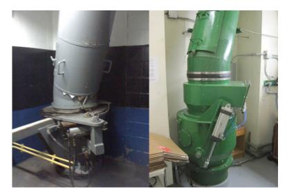
Once the compactor container is full, it is replaced by an empty container that is delivered by a bridge crane, roller-tracks, or other means. Roosevelt Island's facility can store up to 10 containers for transport.
