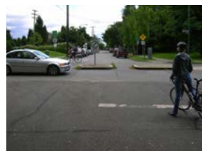
Median Traffic Diverters:
