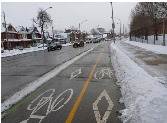
Hamilton, ON: Two-way cycle tracks in Hamilton are routinely cleared of snow using plows (source: Norma Moore)
