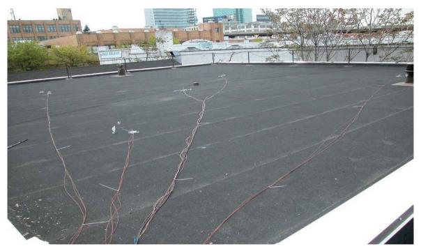
Installation of TI, TM, TT and TA Thermocouples. TI is at the ceiling inside the building. TA is covered by radiation shield.
