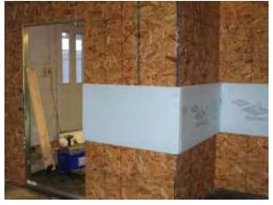
The model process provided a helpful, hands-on means of demonstrating different assembly aspects as they relate to on-the-job issues that may occur with the use of added continuous rigid foam insulation. The model displayed multiple assembly options, allowing contractors to view the inside of the wall cavity in order to examine screw penetration and other aspects of the construction.
