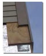
corner, leaving no suitable way to secure a fastener. To address this problem, furring strips, plywood, OSB, metal corners, or other suitable material can be applied over the corners to create a permanent attachment surface. The materials must be wide enough to enable carpenters to secure them to the closest stud. Metal may prove to be the most practical material because its relative thinness compared to wood and
