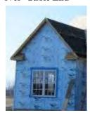
A second option (see Figure 17) is to build the gable end so that the OSB or other sheathing lines up with the foam sheathing to eliminate any transition. This option will likely be more practical with thinner foam insulation. The gable end cannot be offset more than an inch or two, or there will not be a way to attach it to the wall below. As a third alternative, it may be possible to fur -out the gable end.
