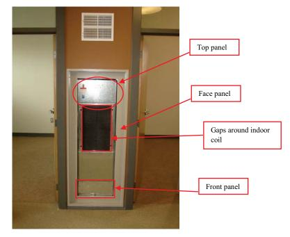
Figure 5-1: General locations of air bypass at site #5
