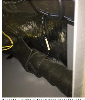
Wires to Symphony thermistor under foam tape insulation
