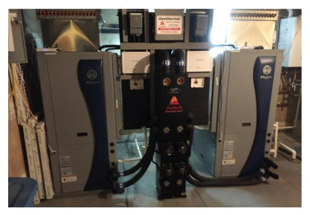
Figure B-1. Two Heat Pumps installed at Niskayuna
