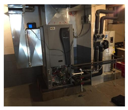
Figure B-5. Heat Pump installed at Akron
