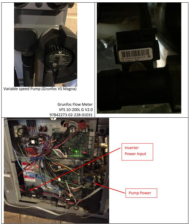
Figure B-6. Controls and Symphony Sensors in the Water Furnace Unit
