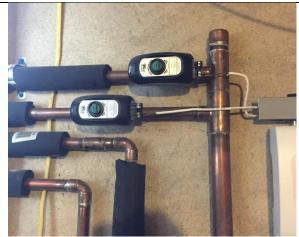
Solenoid Valves controlling HW coils for auxiliary heat
