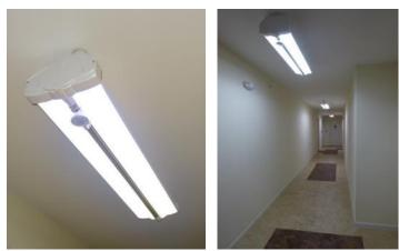
Figure 7. Hallway Lighting with Integral Sensors
