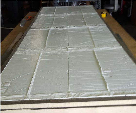
Figure 16. Completed first layer with 1-inch polyisocyanurate at perimeter
