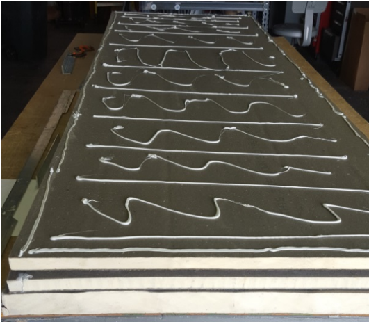
Figure 17. Adhesive applied to top 1-inch polyisocyanurate board
