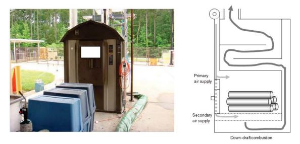
Figure 2. The Three Stage HH Unit and Illustration of a Down-Draft Combustion Unit.
