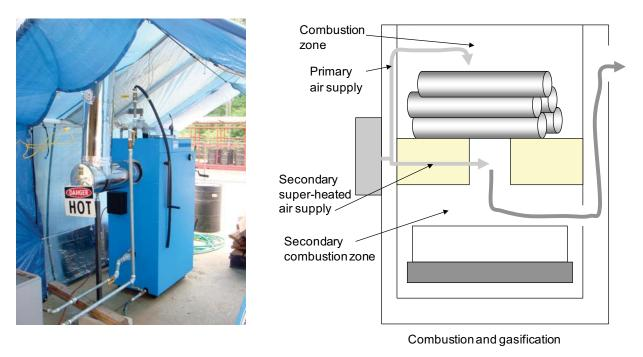
Figure 4. The U.S. Two-Stage, Down-draft Combustion and Gasification Unit Schematic.
