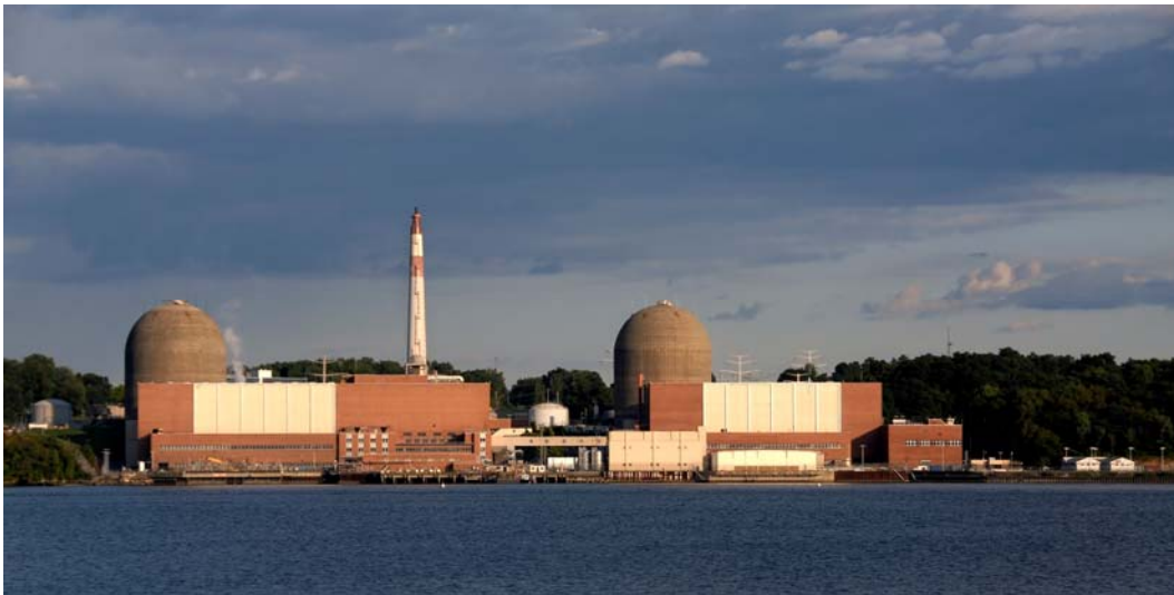
A nuclear power plant on the Hudson River in New York State.
