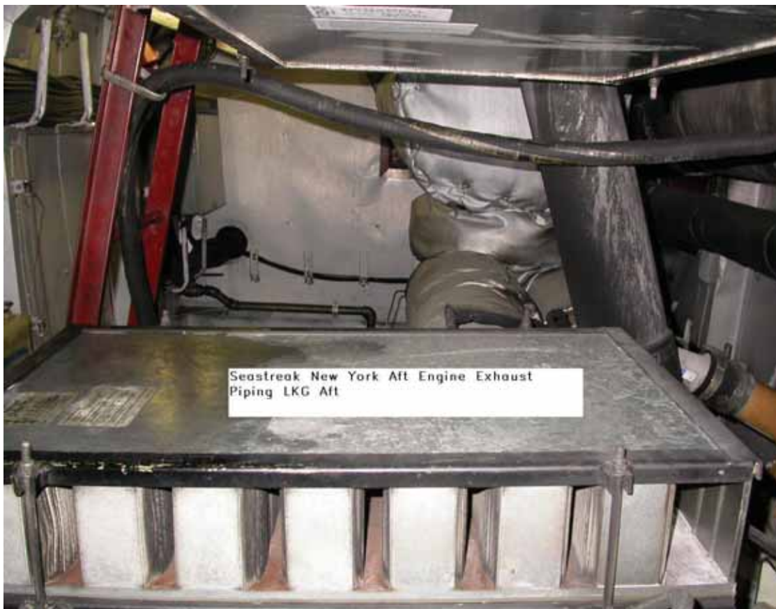
Figure 2.48. MV SEASTREAK NEW YORK sister vessel to MV SEASTREAK WALL STREET Aft Engine.
