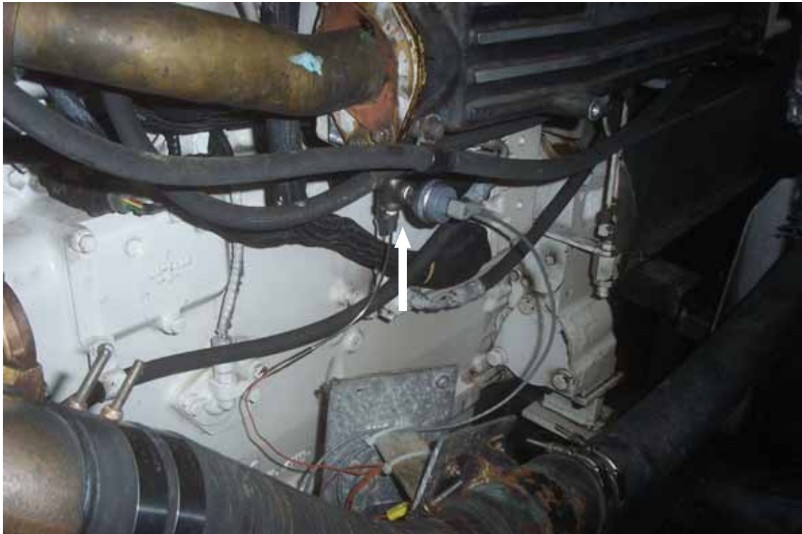
Figure 2.3. Thermocouple and Pressure Sensor Installation.
