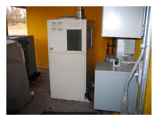
Figure 1-1. Current Installation of Aisin Seiki G60 Cogeneration Unit at Hooligans
