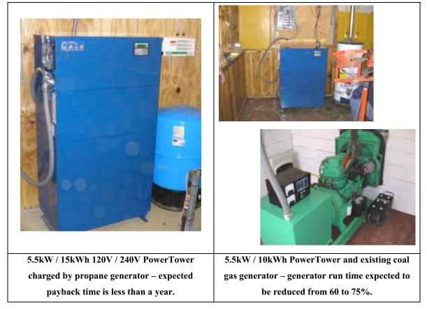
Figure 46: Two off-grid installations with generators – in both cases the generator run time will be reduced by at least 60%
