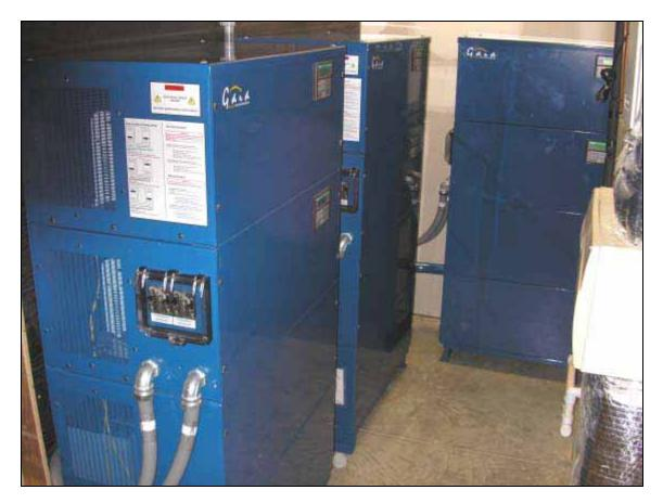
Figure 48: Three 11kW/10kWh PowerTowers are installed for residential backup; the batteries are shared among the three units
