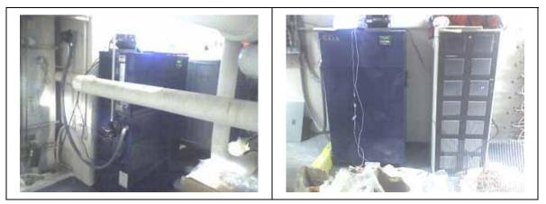
Figure 44: Two PowerTowers at Starwood's Times Square W Hotel providing extended backup and demand reduction for a Motorola and a Nextel repeater station
