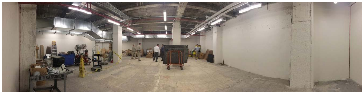
Figure 43. Unused basement space with pre-existing ventilation and fire suppression system
