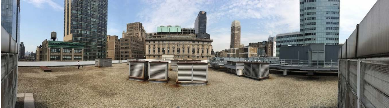
Figure 47. Rooftop space housing existing mechanical equipment
