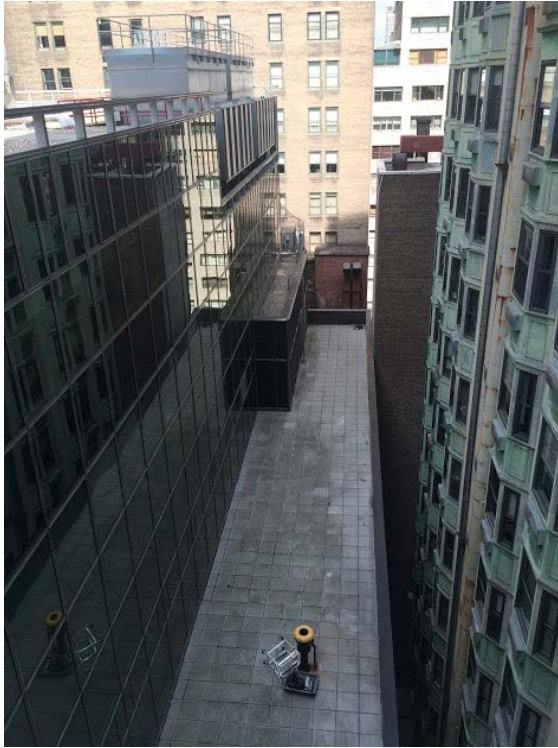
Figure 46. Setback space adjacent to emergency generator room
