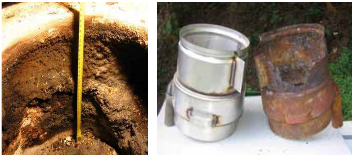
Figure 10-7 corrosive attack of refractory materials after operation with grain (left) and corrosion of metal after straw combustion
