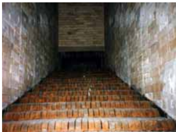
Figure 2-28 Combustion chamber of a moving grate furnace (Polytechnik 2007)
