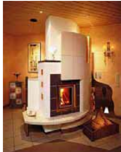
Figure 2-13 Example of a combined tiled stove (Kachelofenverband 2007)
