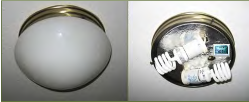
Figure 8: Dome Style Fixture – Remove Dome
