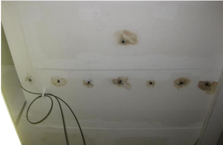
Figure 3-7. Duct Airflow Measurement at Project #1, Energy-Efficiency Program Area
