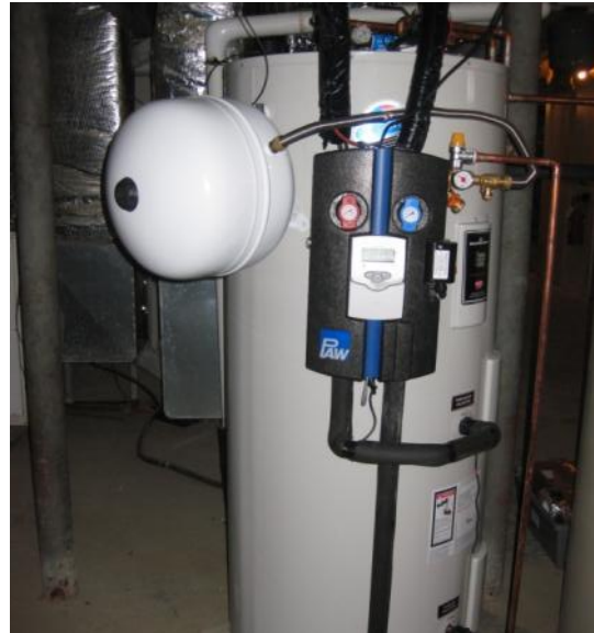
Figure 3-33. Solar Hot Water System Collector Array, Pumping Station, and Preheat Tank, Renewable Energy Program Area
