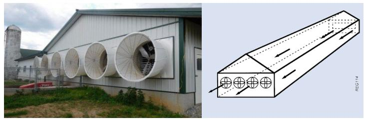
Tunnel Ventilation Design for Enclosed Tie Stall Barn. Photo credit: https://extension.psu.edu/tunnel-ventilation-for-tie-stall-dairy-barns.
