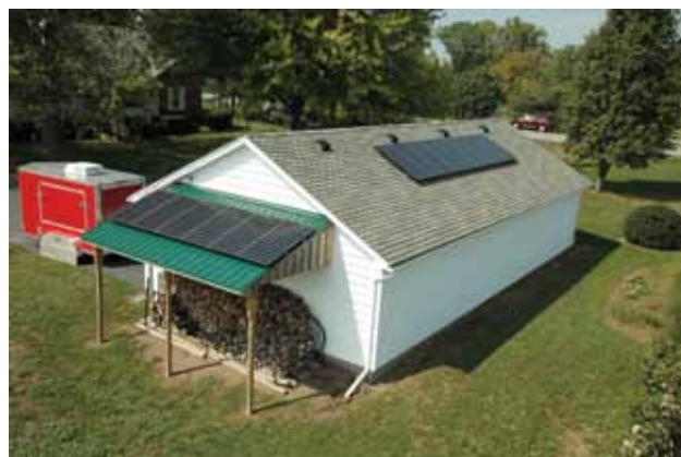
3.6 kW PV System, Lockport, NY
