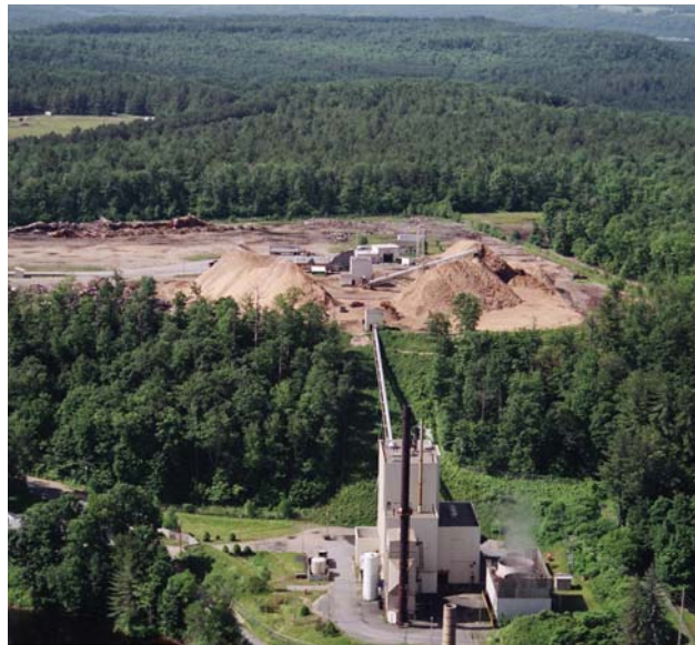
Lyonsdale Biomass Facility, Lewis County
