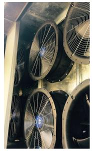
One cell fan wall cooling tower
