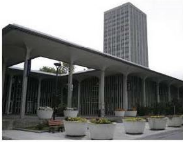
Seneca Hall University at Albany Year Built: 1971 Beds: 82
