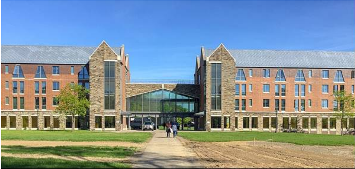
Figure 11. Mews Hall: A 2001 Cornell Dormitory
