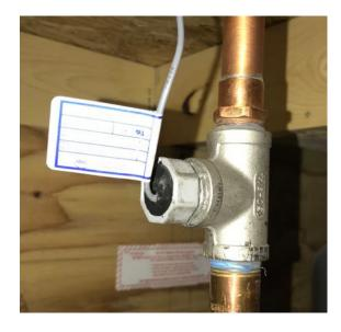
Harwill flow switch in 3/4" SS tee ON at 0.7 gpm OFF at 0.4 gpm
