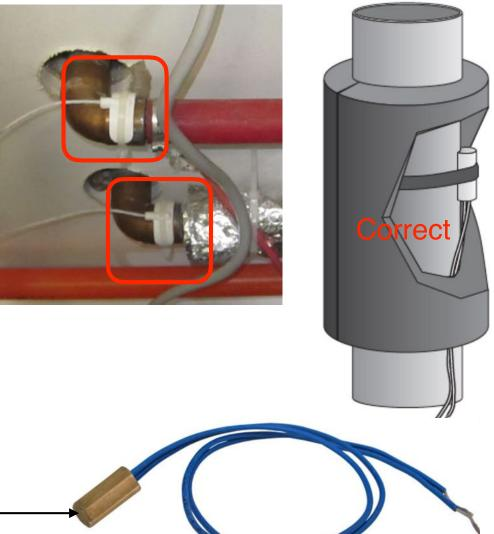
non-insulated surfaced mounted temperature sensors
