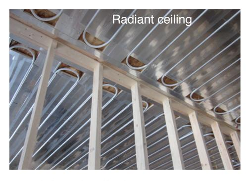
7/16" oriented strand board batt insulation 3/4" foil faced foam insulation 1/2" PEX-AL-PEX tubing, 8" spacing 6" aluminum heat transfer plates, 8" spacing 1/2" drywall
