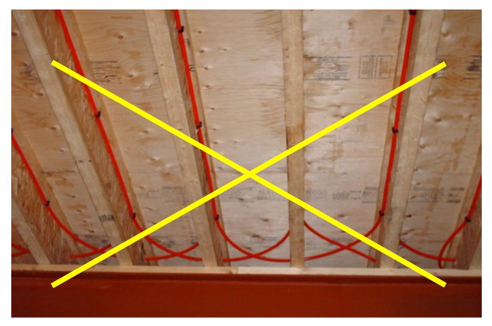
Heat transfer between the water and the upper floor surface is severely restricted!
