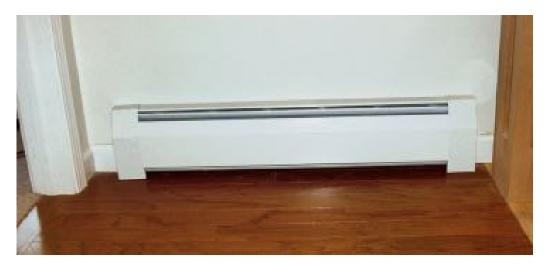
Could add fin-tube length based on lower water temperatures. BUT...
