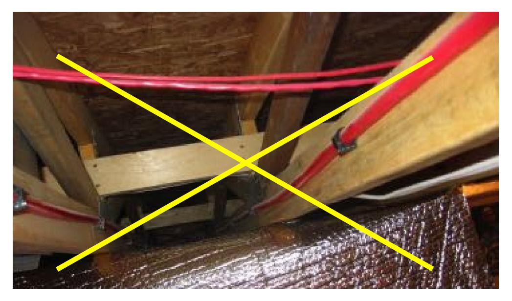
Heat transfer between the water and the upper floor surface is severely restricted!
