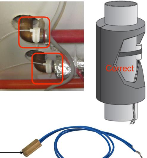
non-insulated surfaced mounted temperature sensors
