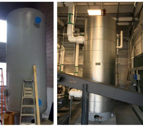
4000 gallon thermal storage tank (before insulation)
