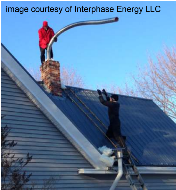
pre-insulated stainless steel liner
