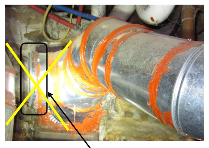
Pellet boiler stack galvanized pipe - no draft regulator
