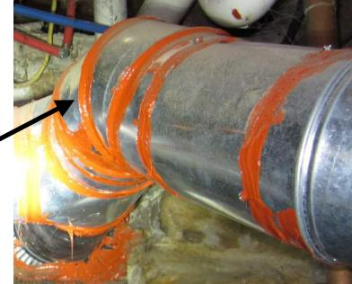
Single wall welded seam stovepipe (22 gauge) can be used.
