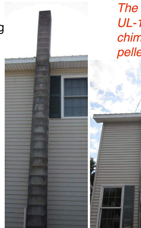
The fix. UL-103 HT chimney for pellet boiler
