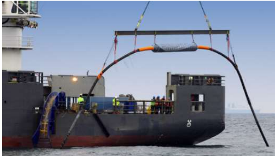
Figure 11.3-11 Vessel Lowering an Offshore Cable Joint Using a Bow
