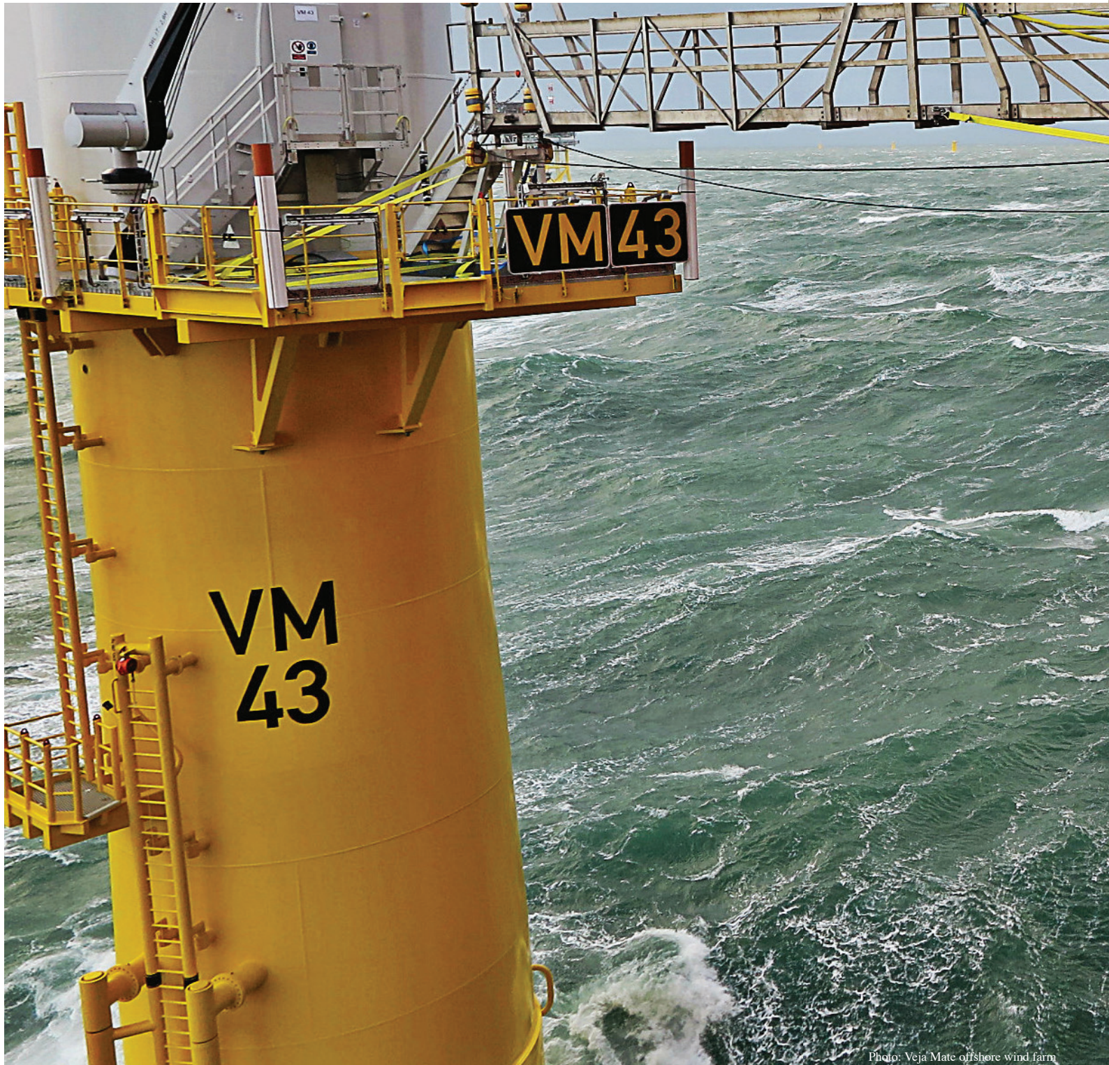
Photo: Veja Mate offshore wind farm
