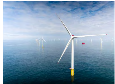
Indicative Offshore Wind Farm: Dudgeon, UK
