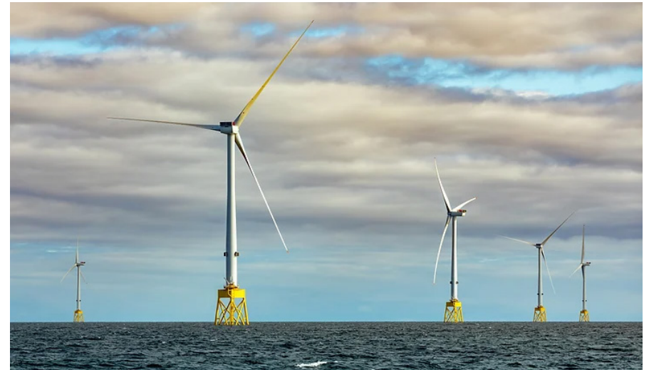
Seagreen's Vestas 10 MW wind turbines
