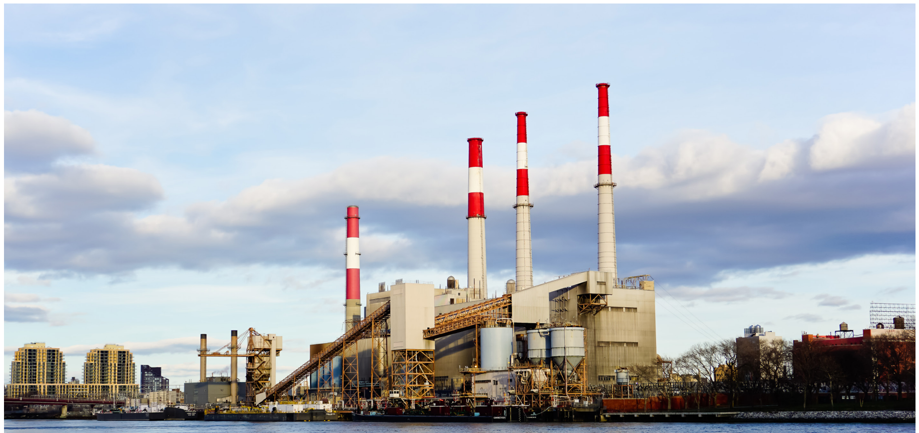
Ravenswood Generating Station, NYC’s largest power plant
