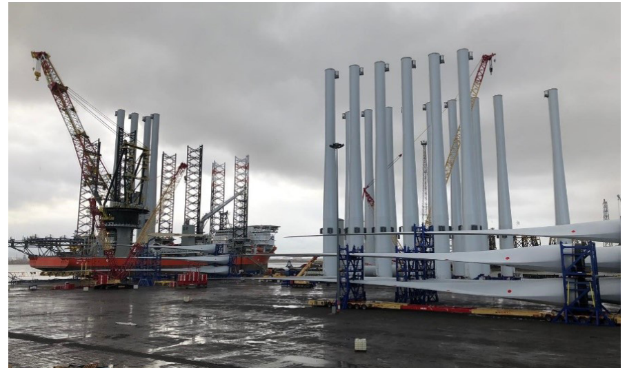
WTG staging and marshaling
