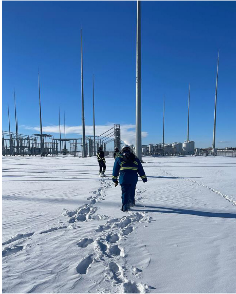
Attentive Energy team at HVDC site visit
