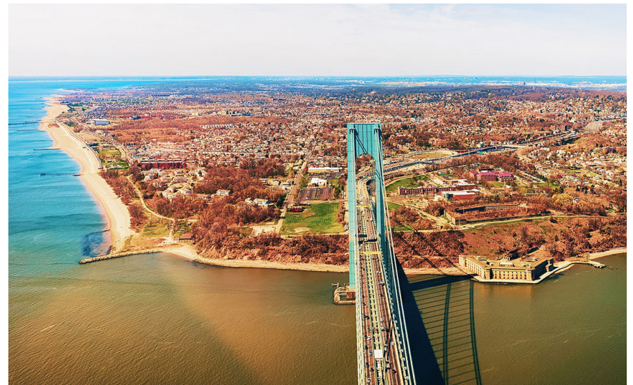
View of Lower Bay from Verrazano-Narrows Bridge
