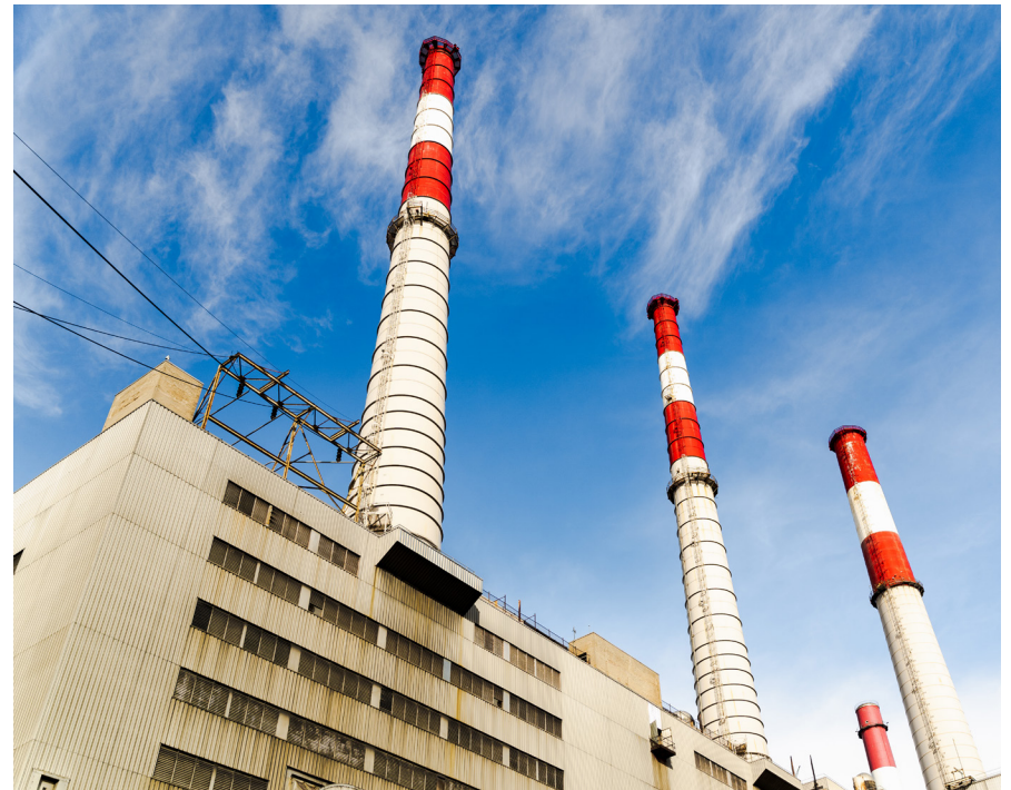
Rise's Ravenswood Generating Station has provided reliable power to New York City for 60 years
