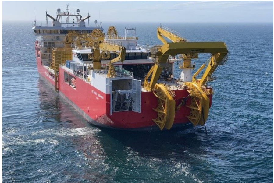
Offshore export cable laying operations
