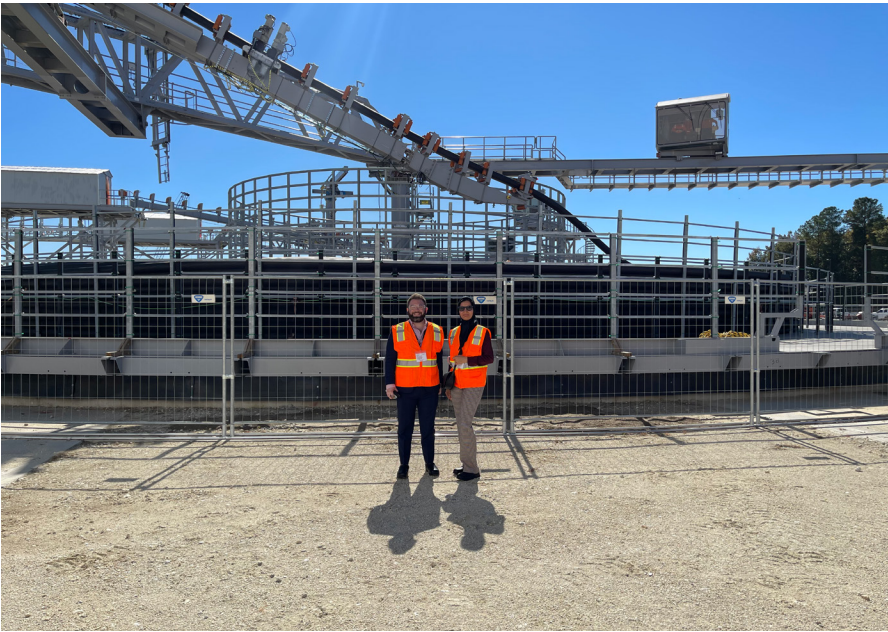
Attentive Energy HVDC cable site visit
