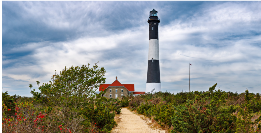
Fire Island lighthouse
