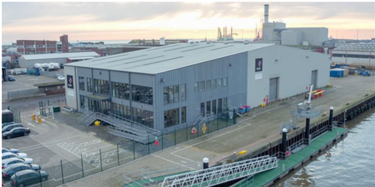
Figure 29: Operations Building for the Dudgeon Offshore Wind Project
