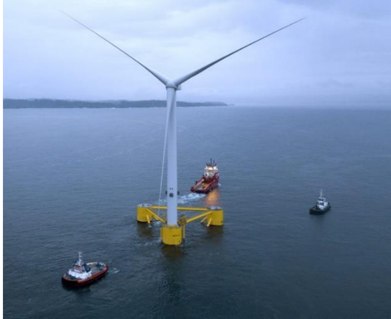
Vestas 8-MW Wind Turbine Being Towed to Station at Wind Float Atlantic
