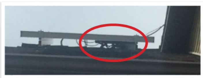
Photo 8 : Source circuit conductors in contact with roof: NEC 338.10, 334.30
