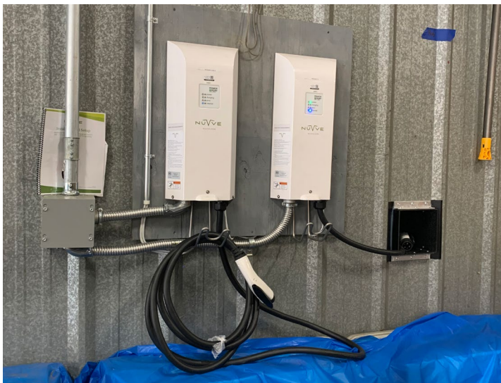
Level 2 chargers can be wall mounted to minimize footprint. An example installed in Croton-Harmon UFSD is mounted in the garage with a cut-through so buses can be charged inside and outside the maintenance garage.
