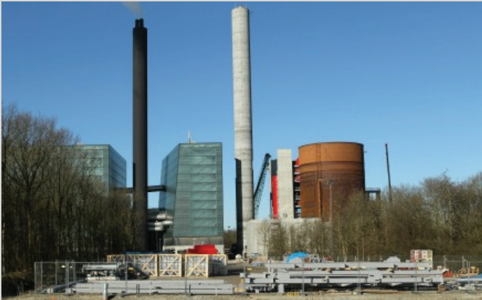
The new Lisbjerg biomass-fueled CHP plant. Photo by Aarhus Kommune.
