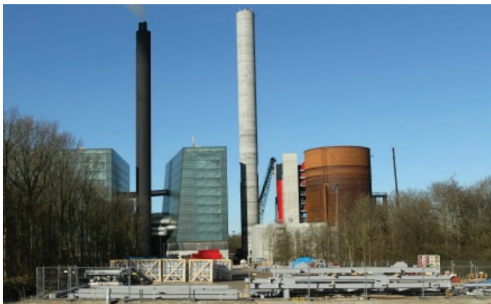
The new Lisbjerg biomass-fueled CHP plant, ready for commissioning. Photo by Aarhus Kommune.
