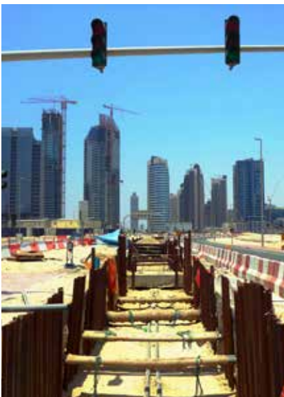
Laying district cooling pipes in Dubai, UAE.
