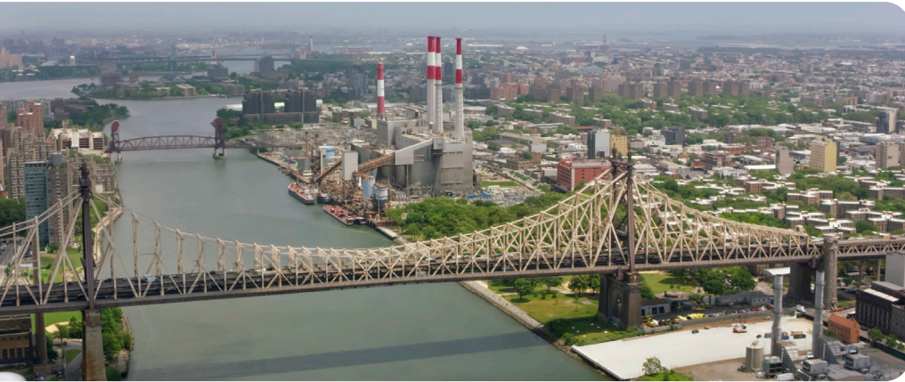
Figure 14-8. Ravenswood Generating Station in Queens.
