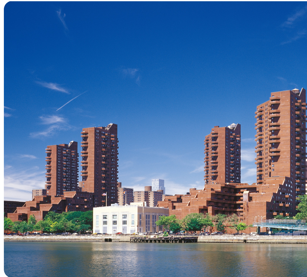
Figure 1-7. The transmission line runs for six miles in the Harlem River before making landfall in the Bronx.
