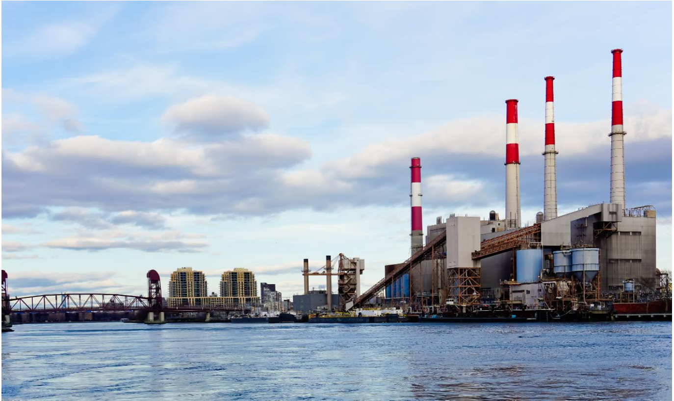
Figure 6. Ravenswood Generating Station
