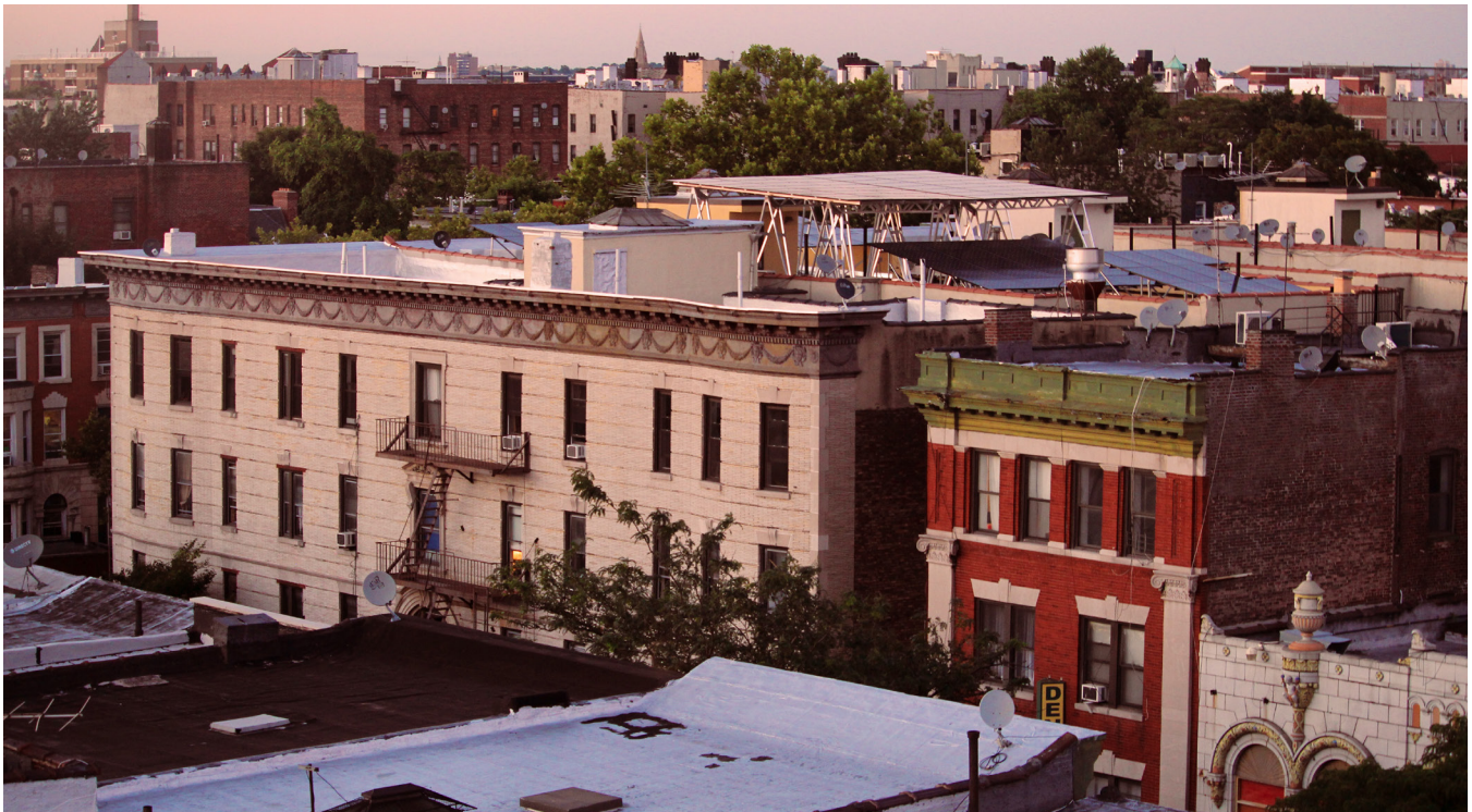
Brooklyn multifamily building with rooftop solar. Photo Credit: Joshua Armstrong
