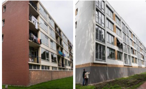
A multifamily building in the Netherlands before (left) and after (right) an Energiesprong retrofit.
