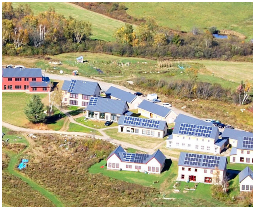
EcoVillage. Photo Source: GO Logic
