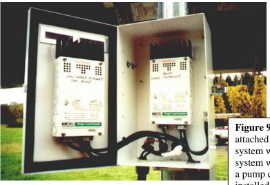
**Figure 9.** A charge controller attached to the array for a system with batteries. For a system without batteries, only a pump controller would be installed.
