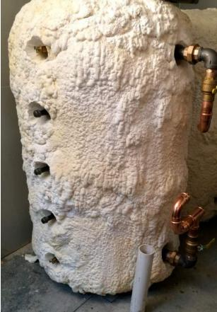
With 4+" of Spray polyurethane insulation + intumescent coating
