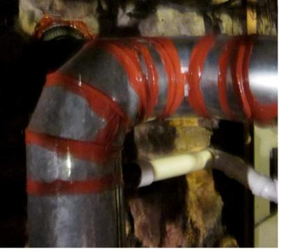
RTV silicone. Will eventually separate from galvanized pipe
