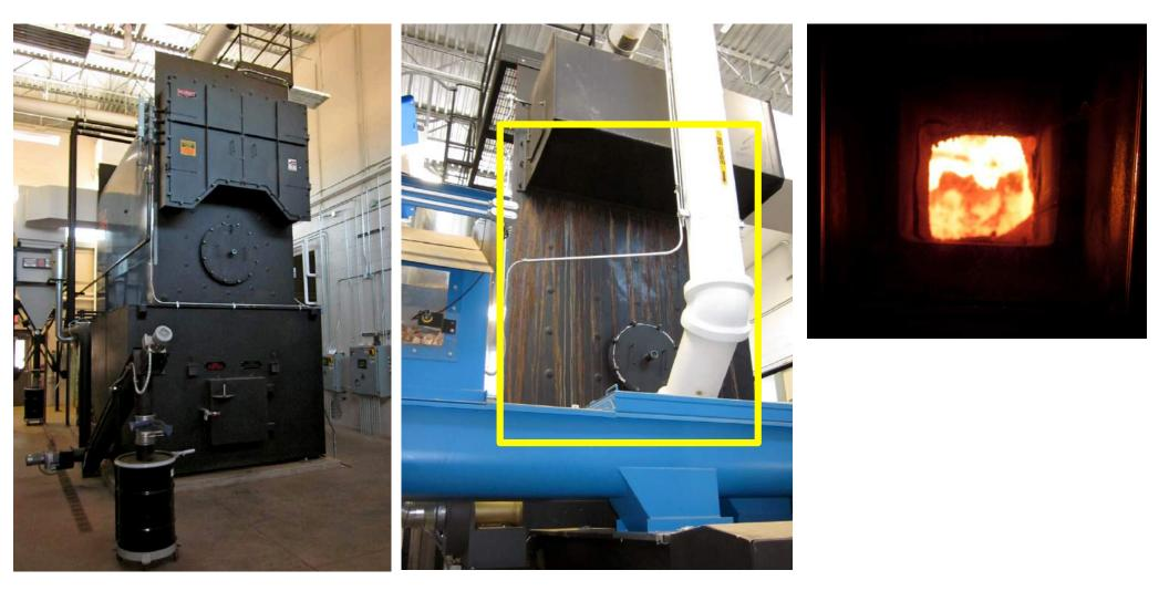
Notice the signs of flue gas condensation on rear boiler plate.
