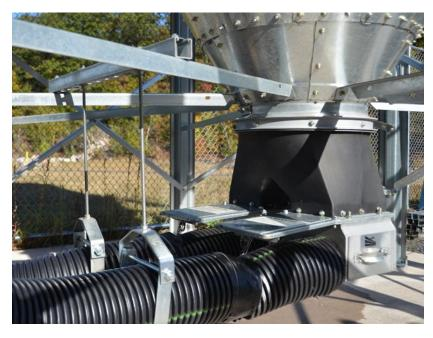
All tubing used for pneumatic pellet transfer should have a ground wire that's attached to the pellet boiler chassis, which itself is connected to an electrical ground. Electrical grounding drains away static electrical charge that could otherwise build up from dust moving along with the high-speed air through the pellet transfer tubing. See the pellet boiler's installation instructions for details on properly grounding the pellet transfer tubing.
