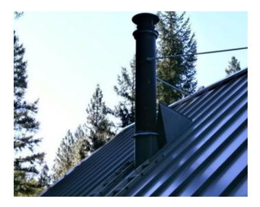
Snow splitters are designed to deflect sliding snow around the chimney and its flashing. Splitters should be made of materials such as aluminum or stainless steel in thickness that can handle substantial force without bending. Snow splitters should also be anchored to building framing using multiple stainless-steel fasteners.
