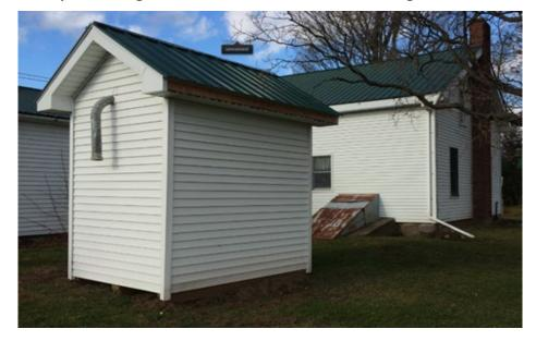
Figure 3-7. Exterior pellet storage bin constructed from common building materials
