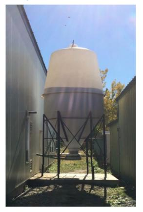
It's also possible to have a pellet storage bin designed to coordinate with building architecture as seen in Figure 3-10.
