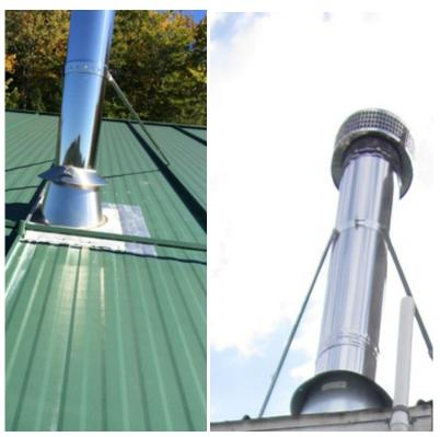
Figure 4-6. Steel bracing of a UL103-HT chimney above a metal roof
