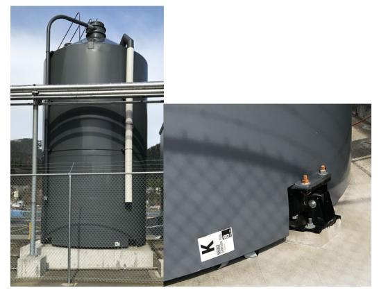
It's important to electrically ground metal pellet bins and silos. A conductor attached to the metal bin or silo is routed to a driven grounding rod, typically adjacent to the pad supporting the bin or silo. Grounding prevents accumulation of static electrical charge that could potentially create a spark. It also helps protect the silo against lightning strikes.
