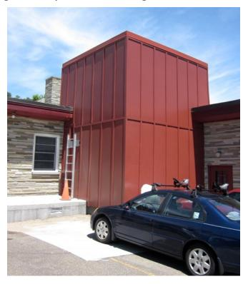
Figure 3-10. Pellet storage bin incorporated into building architecture
