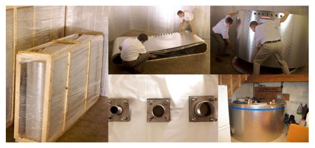
Unpressurized tanks can also accommodate the thermal expansion of the water they contain, assuming that an adequate air space is provided at the top of the tank. This eliminates the need for a separate expansion tank, which is required in systems with pressurized tanks. Another benefit of unpressurized tanks is that they usually cost less on a dollar per gallon basis compared to pressurized tanks.
