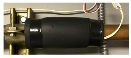
Figure 7-36. Insulation sleeve installed over a small thermistor sensor
