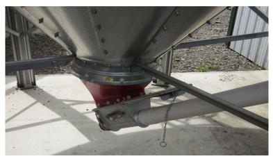
Figure 3-18. Pellet storage silo fitted with a rigid motorized auger assembly
