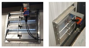
Figure 4-1. Motorized fresh air dampers installed in exterior wall of mechanical room
