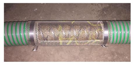
As the pellets pass the screen, fine particles caused by fractured pellets fall through the openings. This reduces fines within the boiler's stoker queue and stoker auger. If a fines screen is used it should be supported above a collection pail. The pail should also be covered to prevent dust emitted from the screen from becoming airborne within the mechanical room. The collection pail should be periodically checked for accumulation and emptied.
