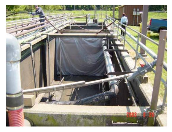
Figure 6-4. Installing Fiberglass Sheeting on the Baffle Wall Face
