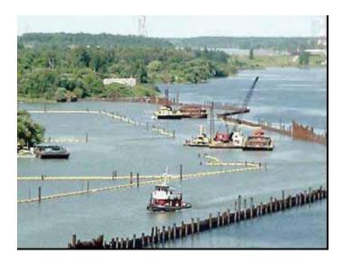
Figure 2-5. Fixed Sheet Piles
