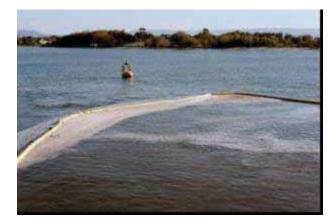
Figure 2-4. Silt Curtains
