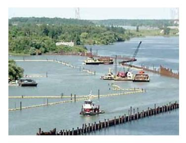
Figure 2-5. Fixed Sheet Piles
