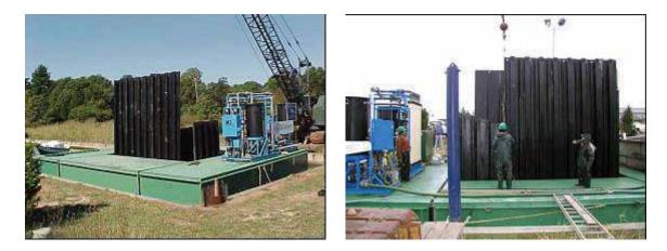
Figure 3-4. Connected Barges with Sheet Deployment
