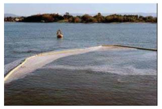
Figure 2-4. Silt Curtains
