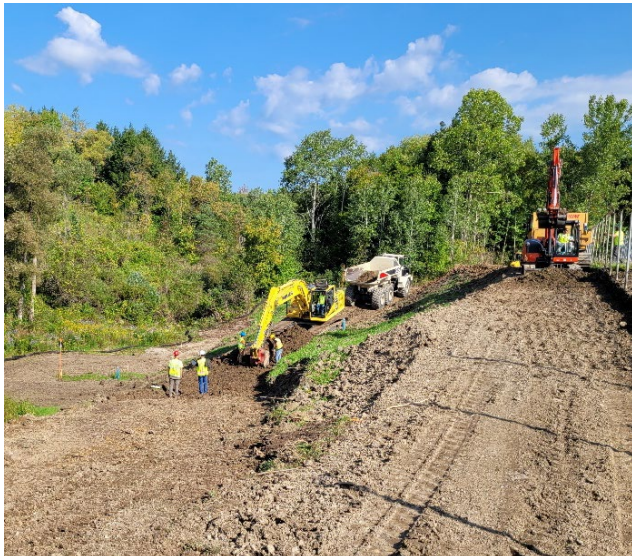
Figure 4-3. Loose soil removal from the North Slope
