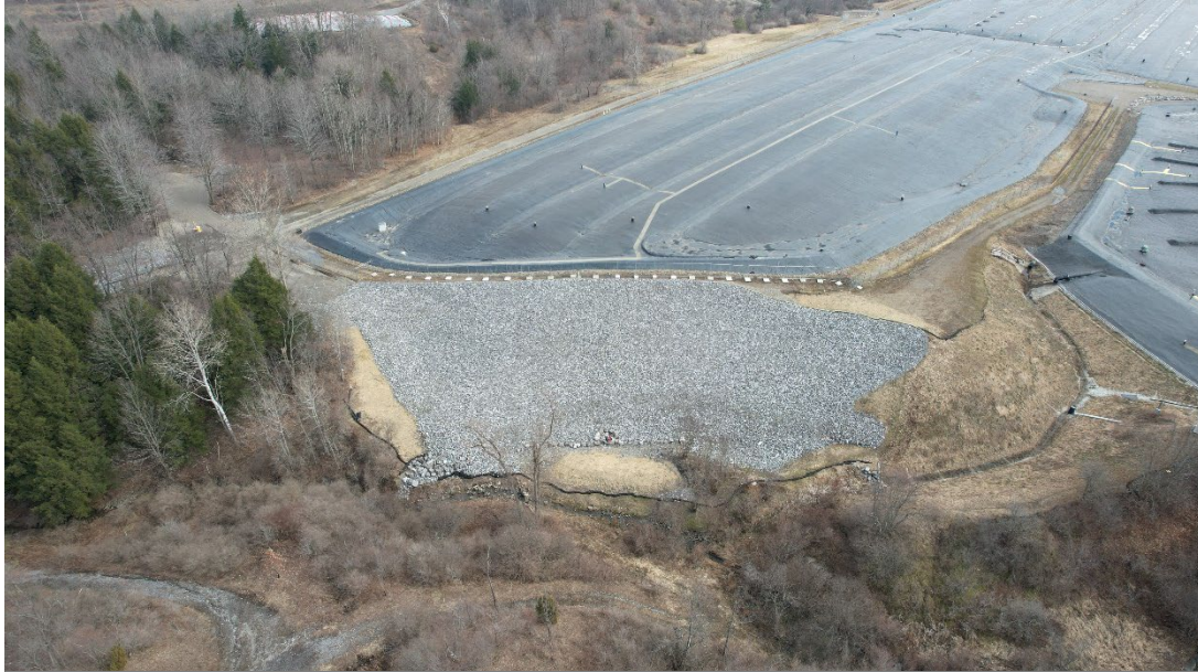
Figure 4-5. Aerial view of the completed North Slope Stabilization Project
